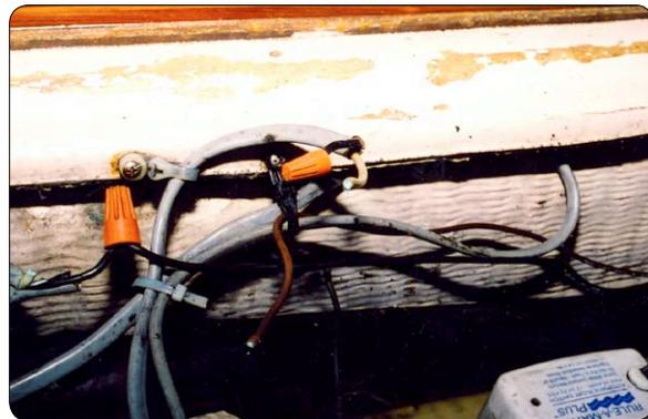
**Wire nuts like these have no place on a boat. Designed for solid core wire, which also should never be used aboard, wire nuts cut into stranded wire, damaging the connection and potentially causing a fire.**
